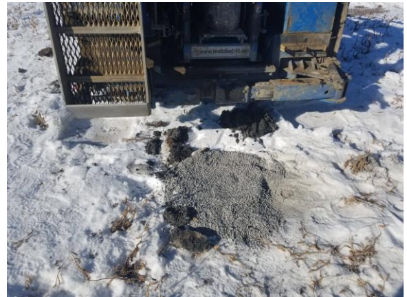
Photo #4 View of completed sealing at borehole 1358-14 (1).
