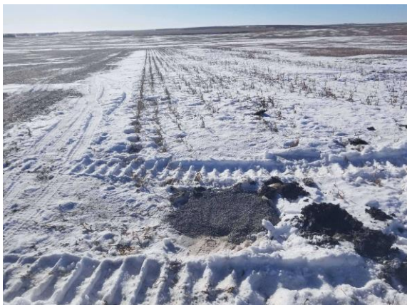
Photo #5 View of completed sealing at borehole 1358-14 (1).
