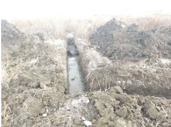
Photo #11 View of water filling the excavation trenches.
