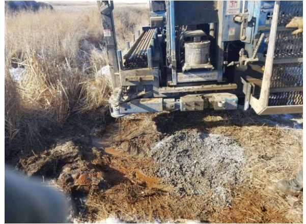
Photo #8 Sealing completion at borehole 1358-14 (2).
