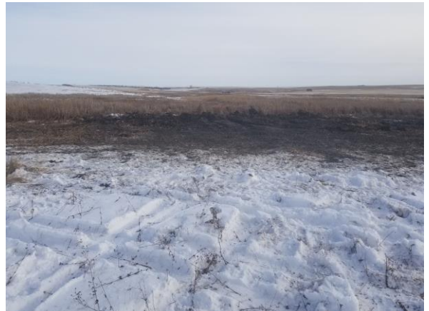
Photo #12 View of leveled excavation area due to cave in and request of the landowner.
