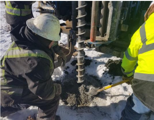
Photo #3 View at borehole 1358-14 (1) backfilling with bentonite pellets.
